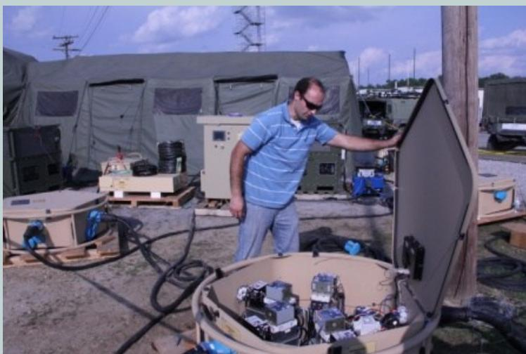
**CERDEC demonstrated a proof of concept for a smart grid that could support tactical operations this summer at its integrated capabilities test-bed at Fort Dix, N.J. (Photo by Spc. Robert Porter/Released)**
